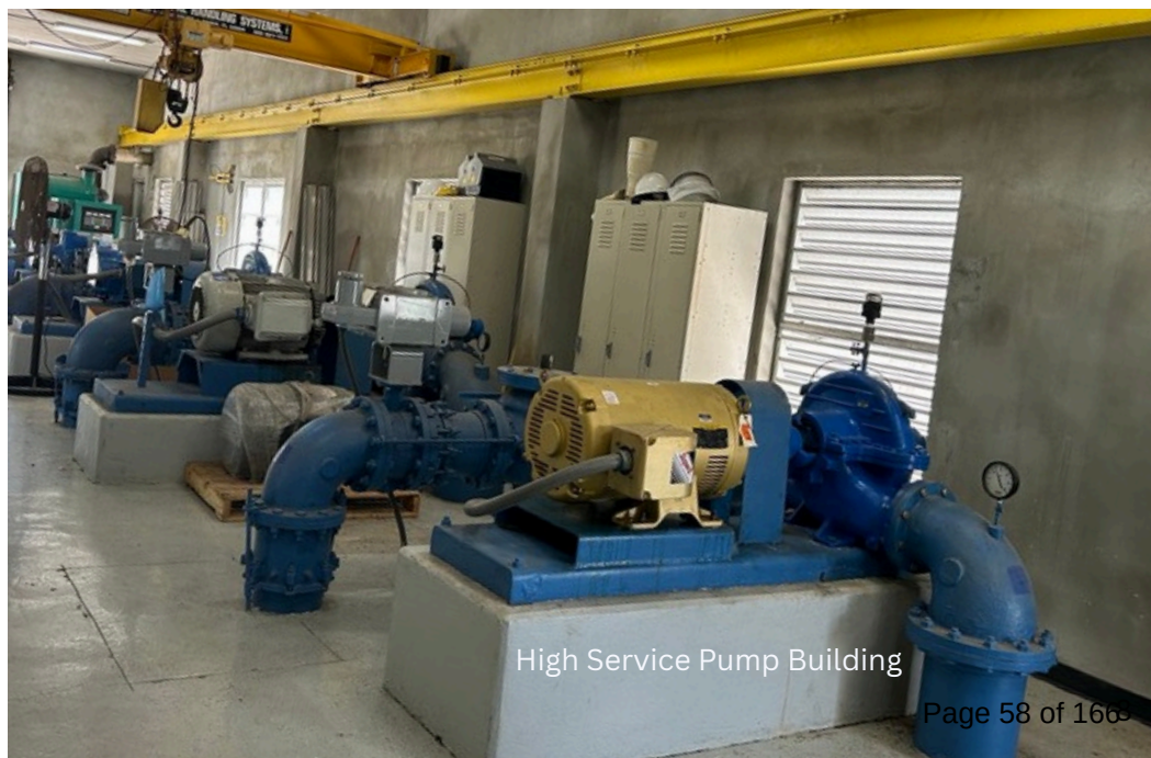
South Water Treatment Plant
